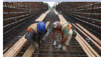
Work continues on the 6.6-mile Expo Transit Corridor extension.
